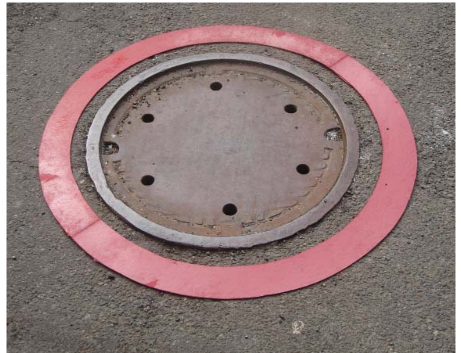
Pavement markings highlight street features
